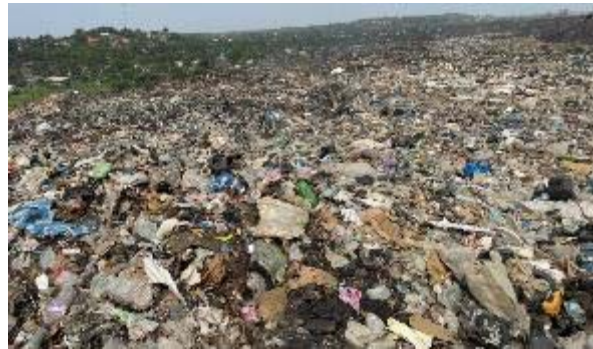
Figure 13. Exposed Waste on Cell 0
