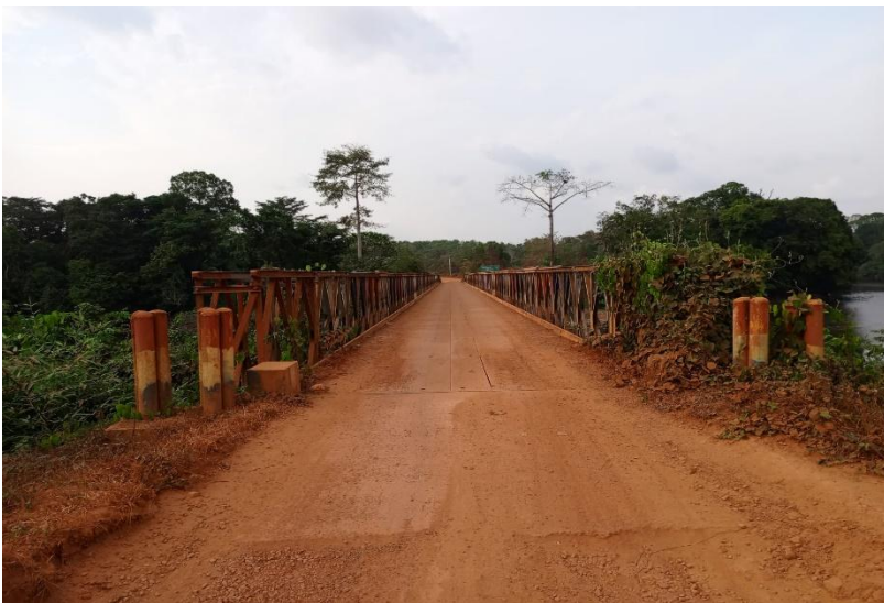
Timbo River Bridge
